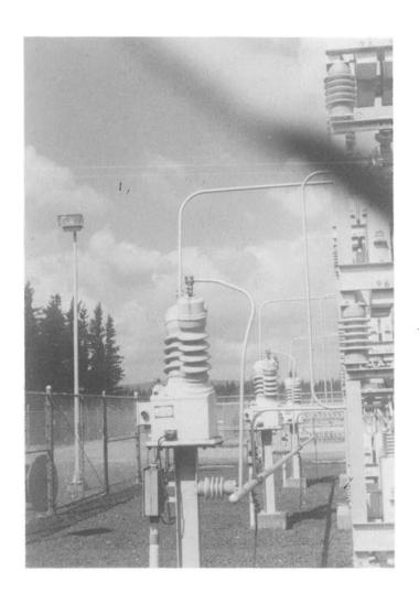
Figure 23: 35 kV PTs Measuring Tap Voltages
