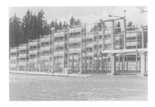
Figure 2: 500 kV Grounded-Wye Shunt Capacitor Bank
