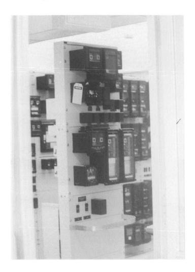
Figure 20: Original Capacitor Control and Protection Panel
