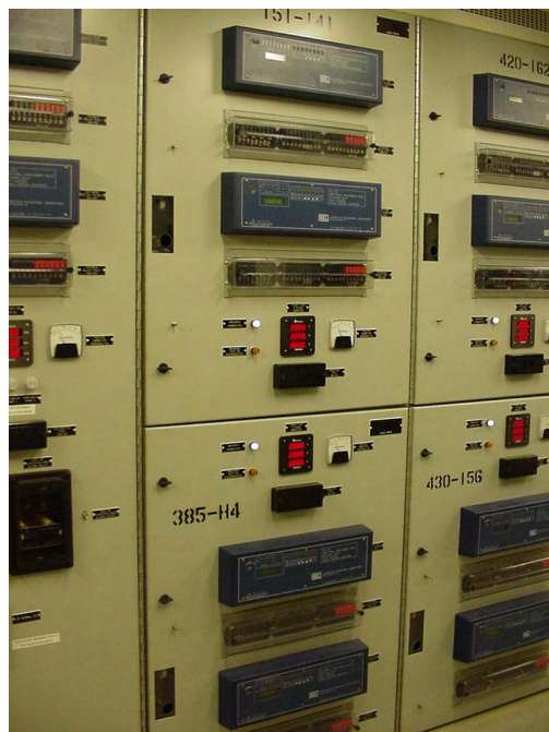
Figure 9 Dual Feeder Protection
