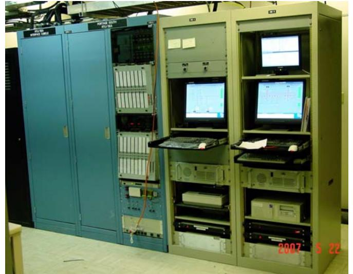
Fig. 5. Standard Manitoba Hydro RTU and HMI Installation
