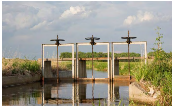
Fig. 1. Conventional Open Channel Flow Control System
